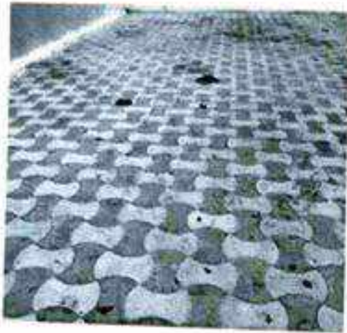
Paving stone installed in campus
