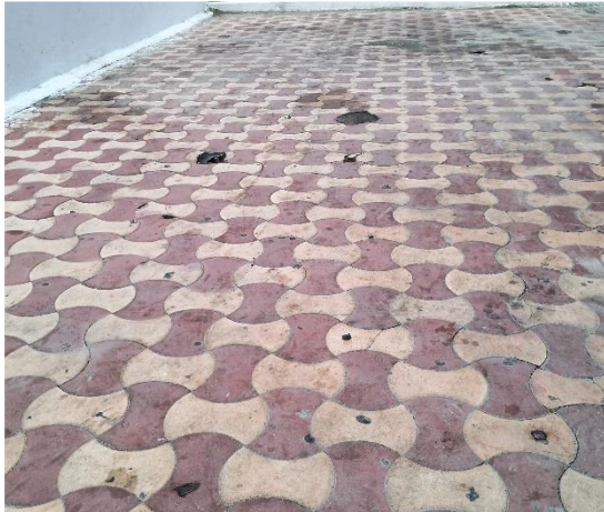
Paving stone installed in campus
